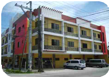
Dormitory front figure
