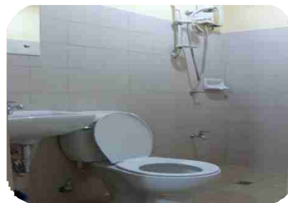
Bathroom each room
